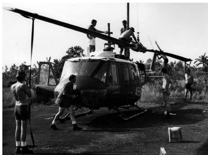
Servicing an Iroquois of No. 5 Squadron during an exercise somewhere in Australia. Source: RAAF Museum
