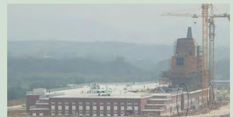
BELOW Dalian mock-up, you can see the jet on the deck and the encircled gaps for deck edge elevators.
